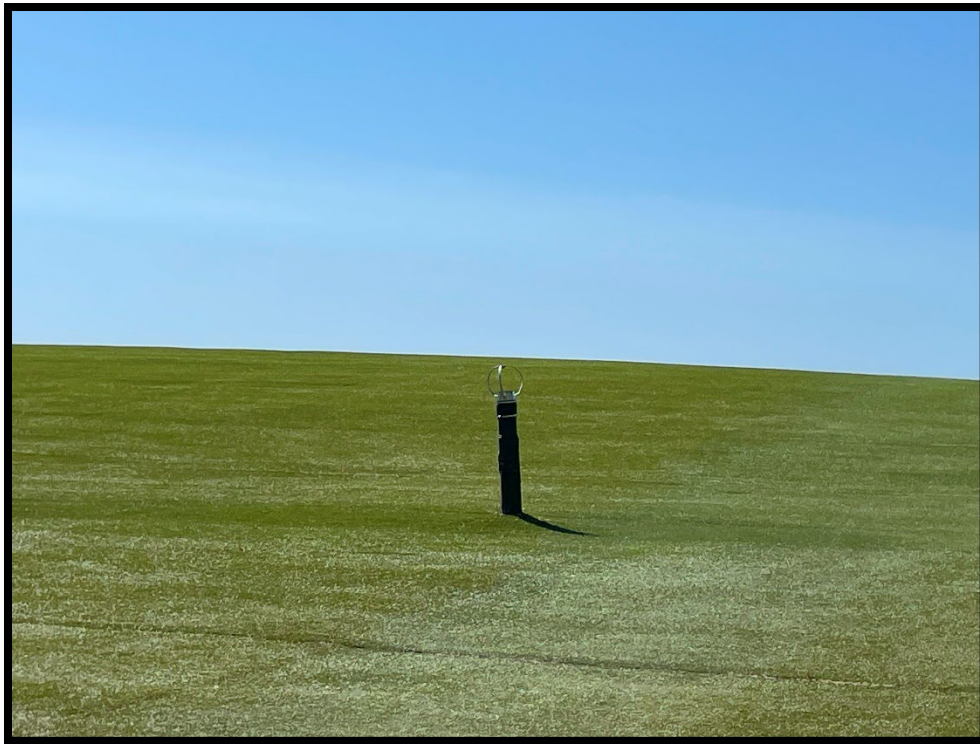
Photograph 1: View of detached turbine vent near LCS-6.
