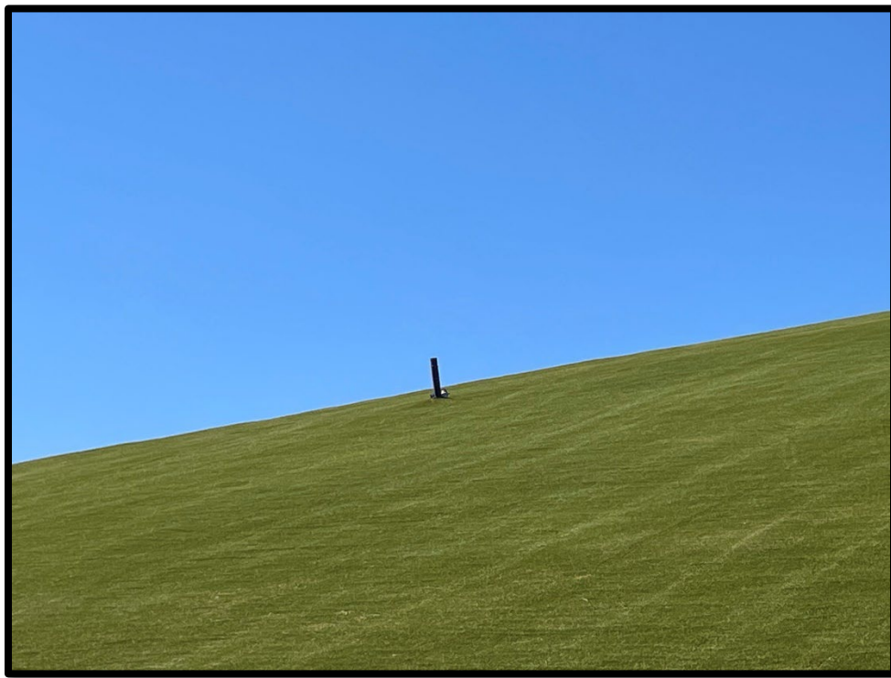
Photograph 2: View of detached turbine vent near LCS-8.
