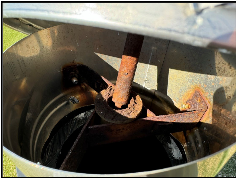
Photograph 4: View of damaged turbine vent on north side of Area 1-2.
